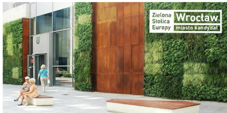
Figure 5. The green façade of the Municipal Office building at Świdnicka Street.
