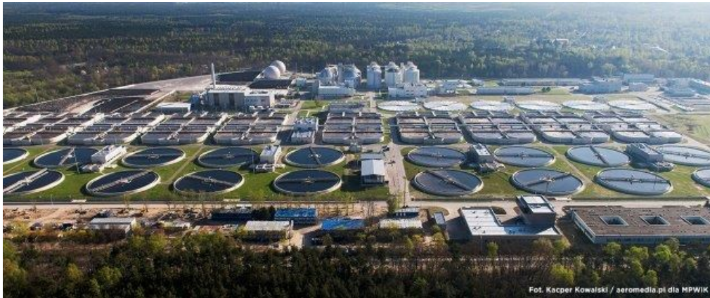
Figure 2. Czajka Wastewater Treatment Plant in Warsaw - an example of eco-innovation.
