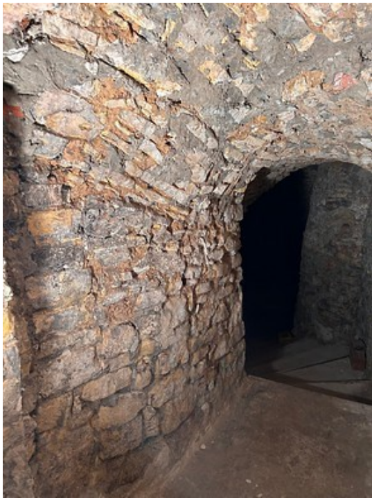
Figure 14, 15. Cellar room with barrel vault.
