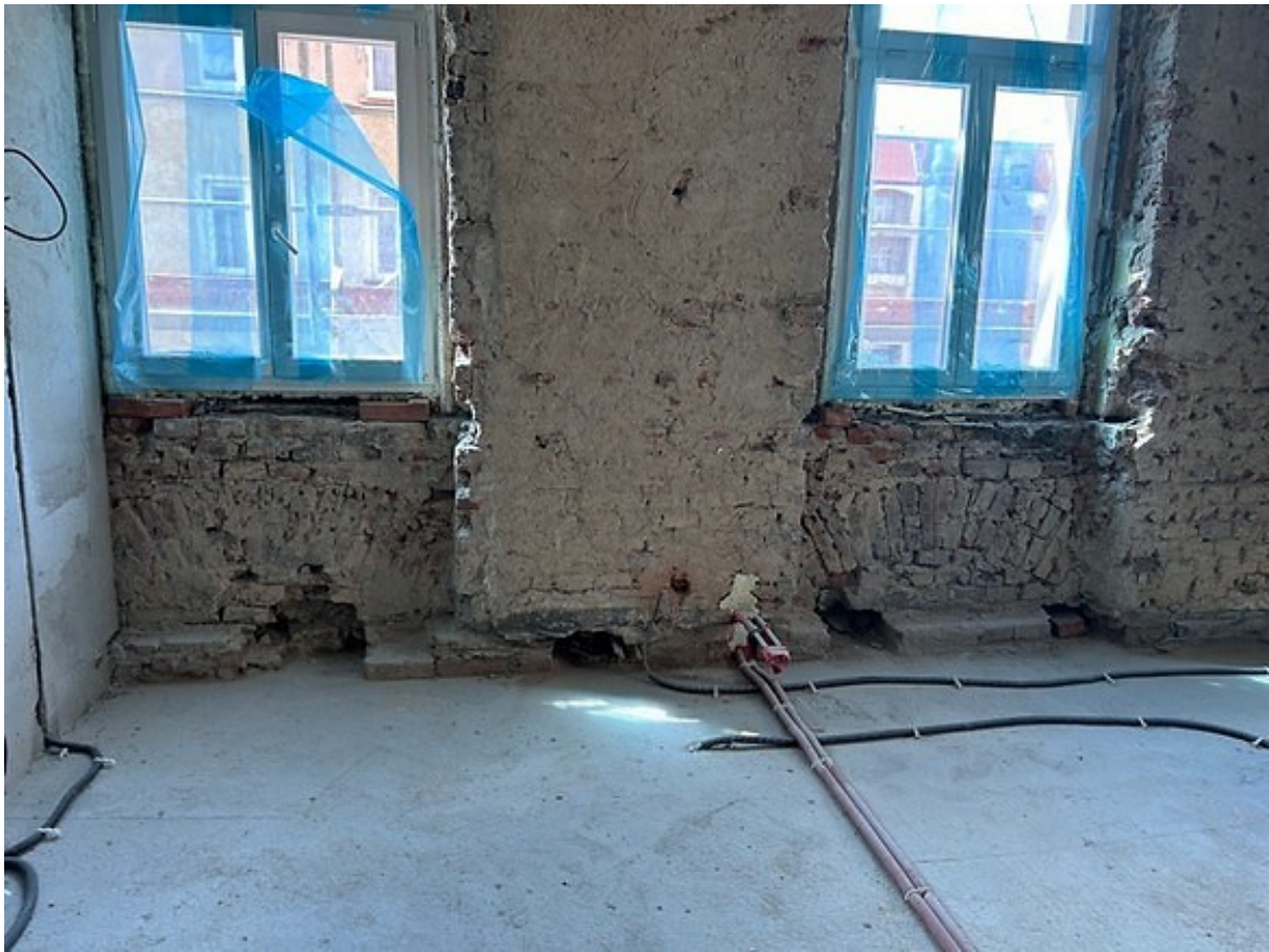
Figure 18. Visible window lintels on the second floor.
