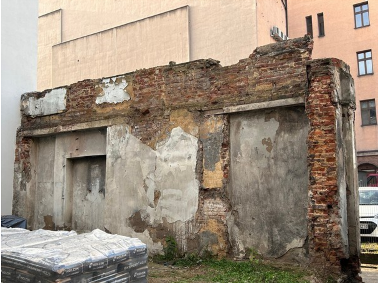
Figure 13. View from the courtyard: clear phases of subsequent transformations of the ground floor zone, identified in archival documentation (1860, 1900, 2020).
