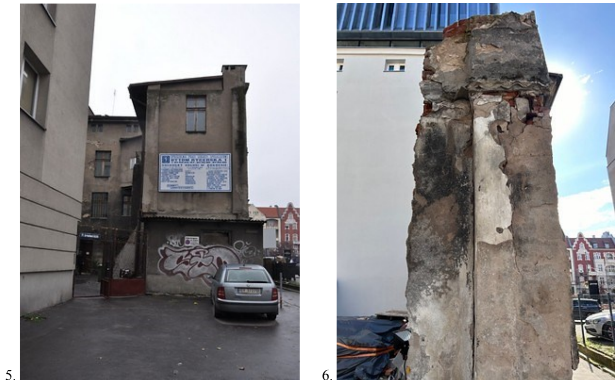
Figure 5, 6. View of the annex building before demolition in 2021 and its condition in 2024.
