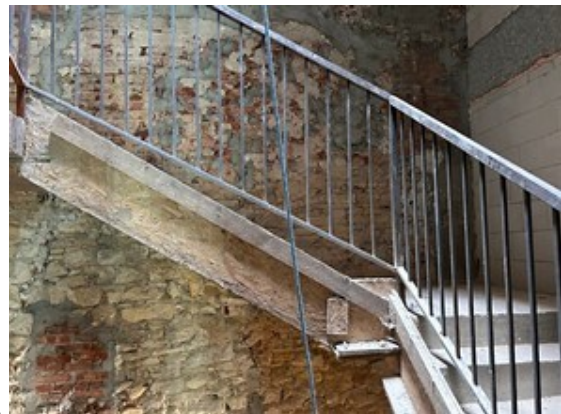
Figure 9, 10. View of the wall on the 1st floor and a fragment of the wall near the staircase, with brickwork and brick inserts visible.
