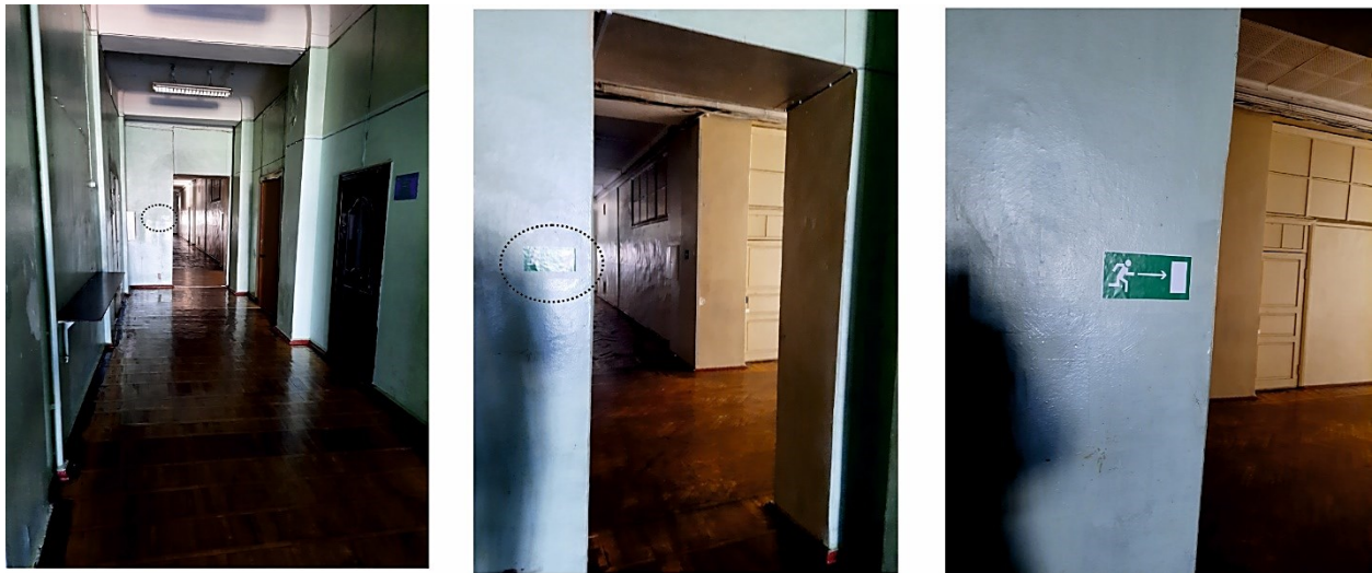
Figure 5. The sign of emergency exit from different distances - 5, 2.5, and 1.5 meters. The glare is on sign surface in a dark corridor from rays of natural light.
