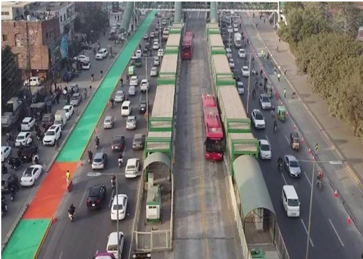
Figure 12. Construction of Bike Lanes along with a dedicated metro bus lane in Lahore.
