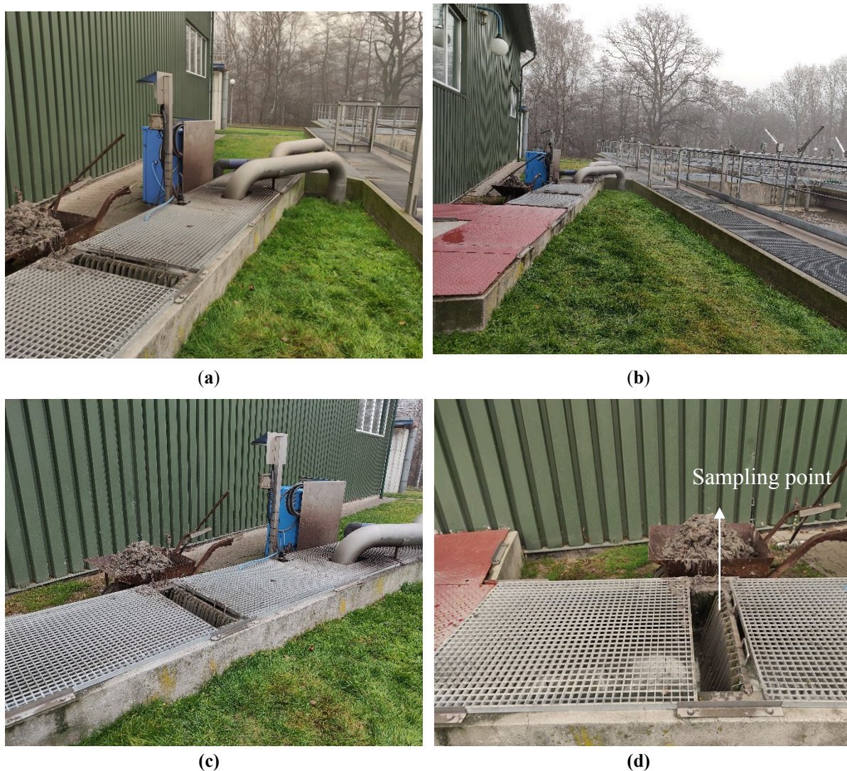
Figure 2. Urban waste water sampling location (a)(b) Mechanical grating station and wastewater inlet to biological reactors; (c)(d) Grating stand - mechanical part of the treatment plant.
