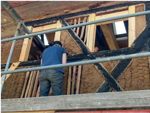
Figure 2. Students weaving straw and clay infill between timber elements using the Lehmwickel technique. (Photo: E. Rdzawska-Augustin, 2022)
