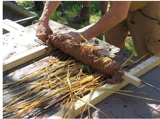
Figure 3. Straw-clay blocks formed and dried on site before being placed into timber frames. (Photo: K. Gerlic, 2024)
