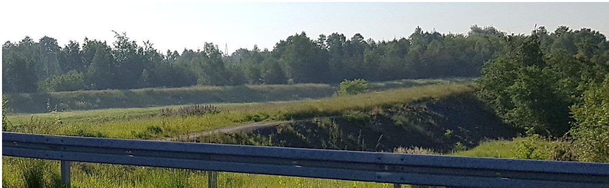
Figure 2. River embankments built as part of the removal of 'mining damage'.
