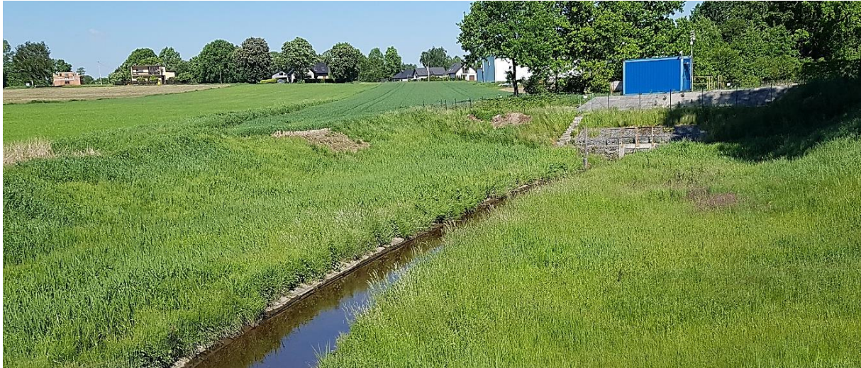
Figure 3. Intake of stream waters in the lower floodplain by the pumping station (view toward the NW) Source: internal materials of SRK S.A
