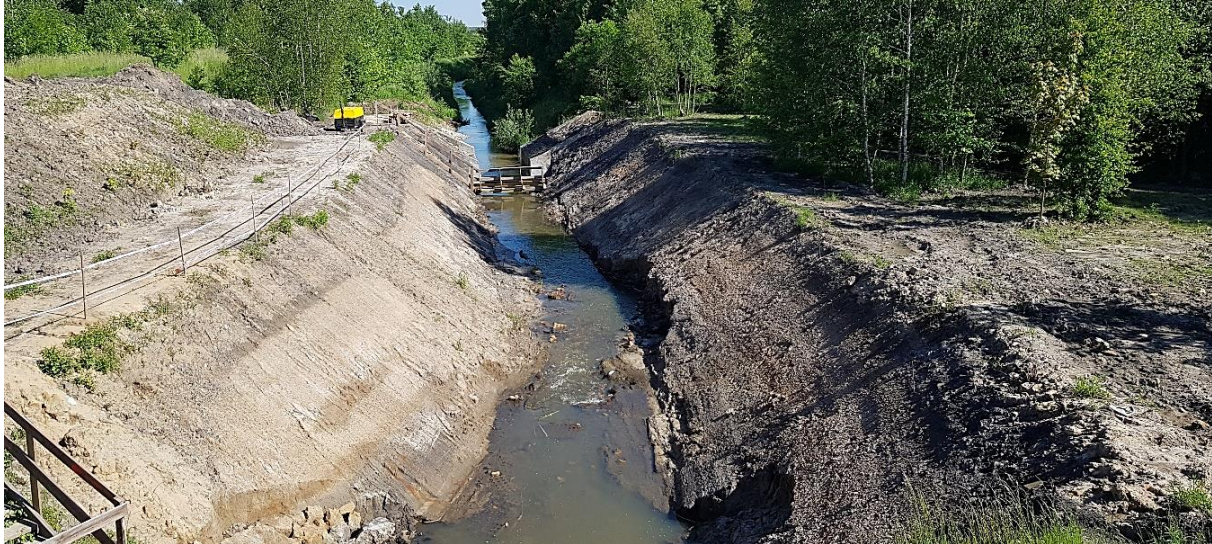
Figure 5. Widening and deepening of the stream bed with a change in the shoreline.
