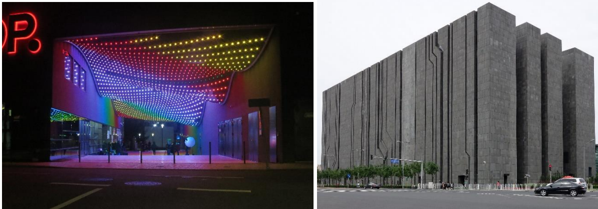
Figure 4. A – World Conference Center Bonn, an example of emphasising the location; a passage. Source: photos by author. B - Digital Beijing Building, (Pei Zhu, 2007) Beijing, China.
