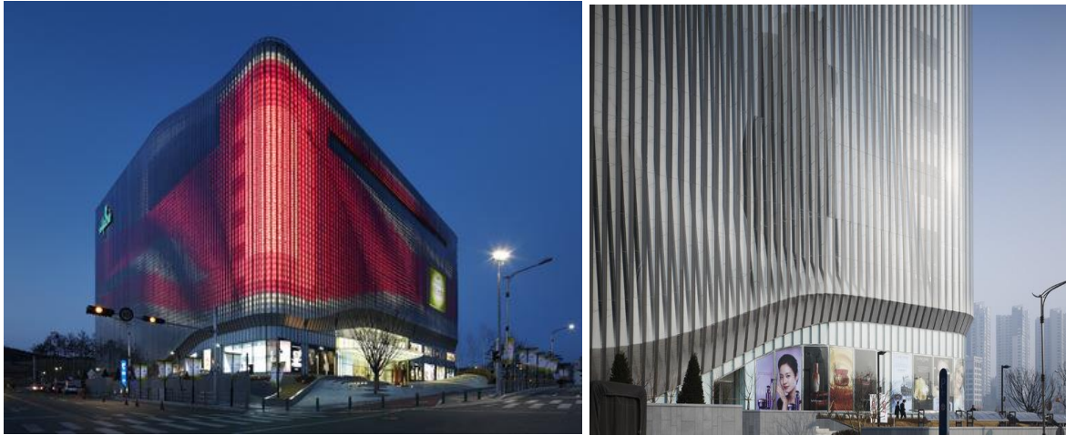
Figure 7. Galleria Centercity (Unstudio, 2010) Cheonan, Korea: A – The façade at night; B – A piece of the façade in daytime, moiré patterns.
