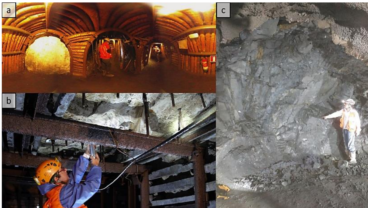
Figure 2. Mines visited for this project: a) 360 panorama in lignite galleries, Utrillas Spain, b) rock mass characterization in Experimental Mine 'Barbara' (Mikołów, Poland) c) fracture and RMR-Q index determination in advancing front in a tunnel, Mine School El Bierzo (Spain).
