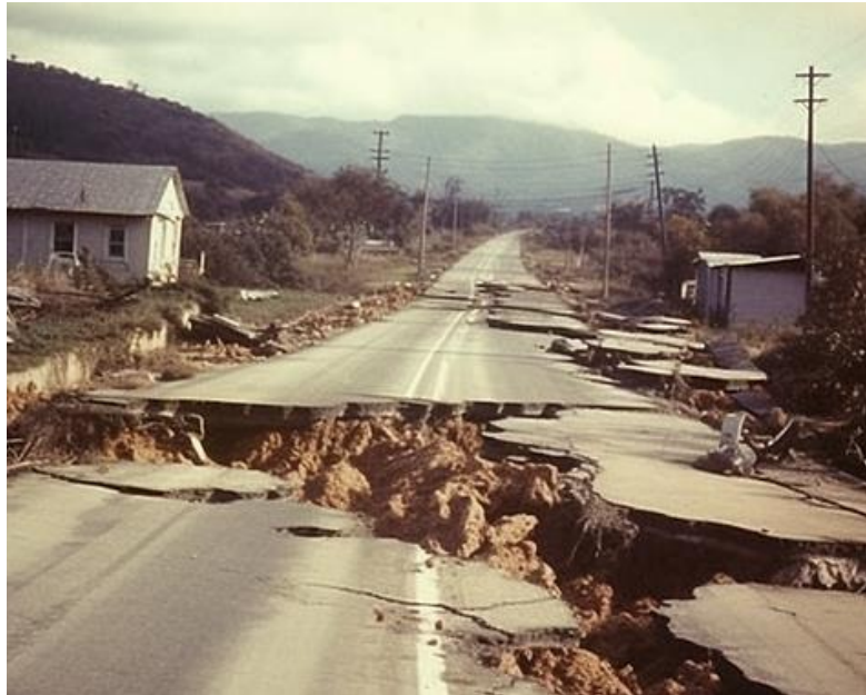
Figure 5. Soil, foundations and safety of facilities in construction.
