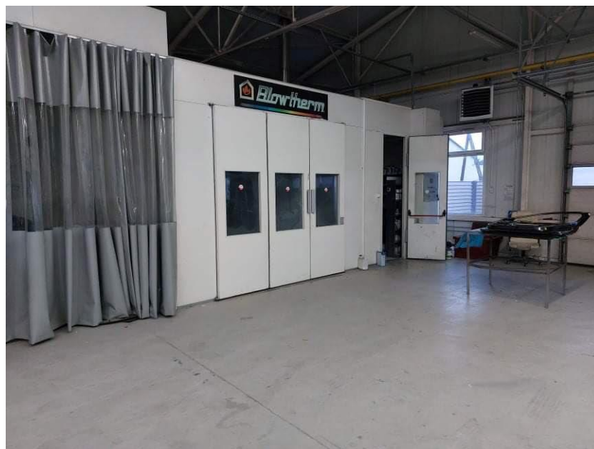
Figure 5. Car Preparation Zone for Painting.
