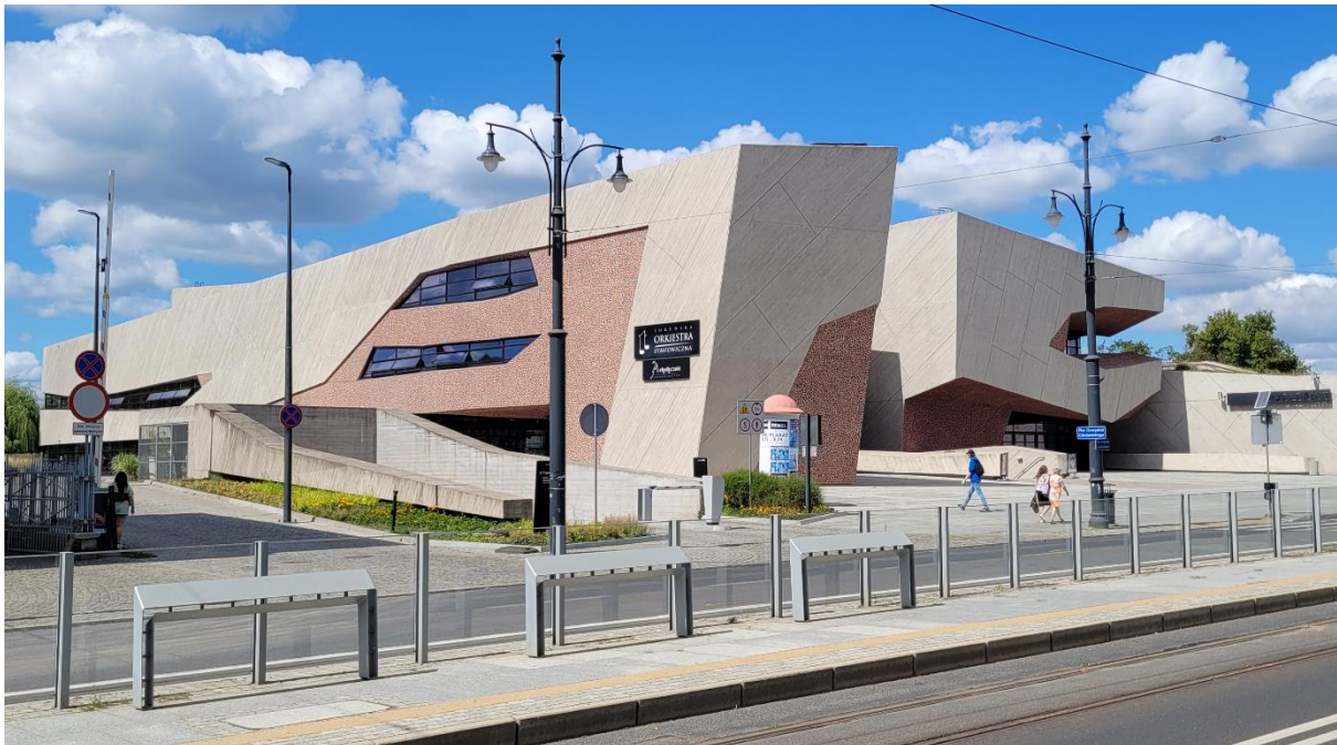
Figure 4. The CKK Jordanki building at Aleja Solidarności, in the northern vicinity of the old town of Toruń. Design: Fernando Menis architect with an international team.
