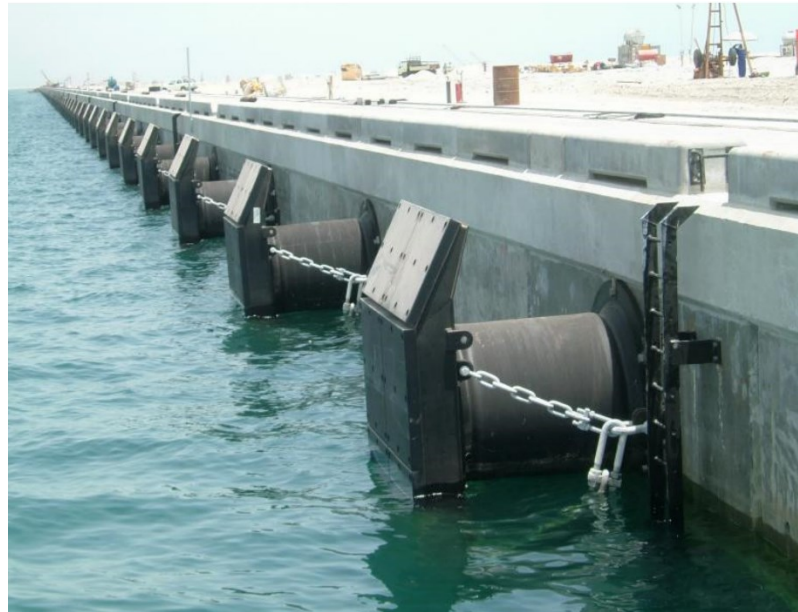
Figure 1. Applications for superduplex stainless steel in seawater: Fasteners for rubber dock fenders (part b) (Francis, Burne, 2021).
