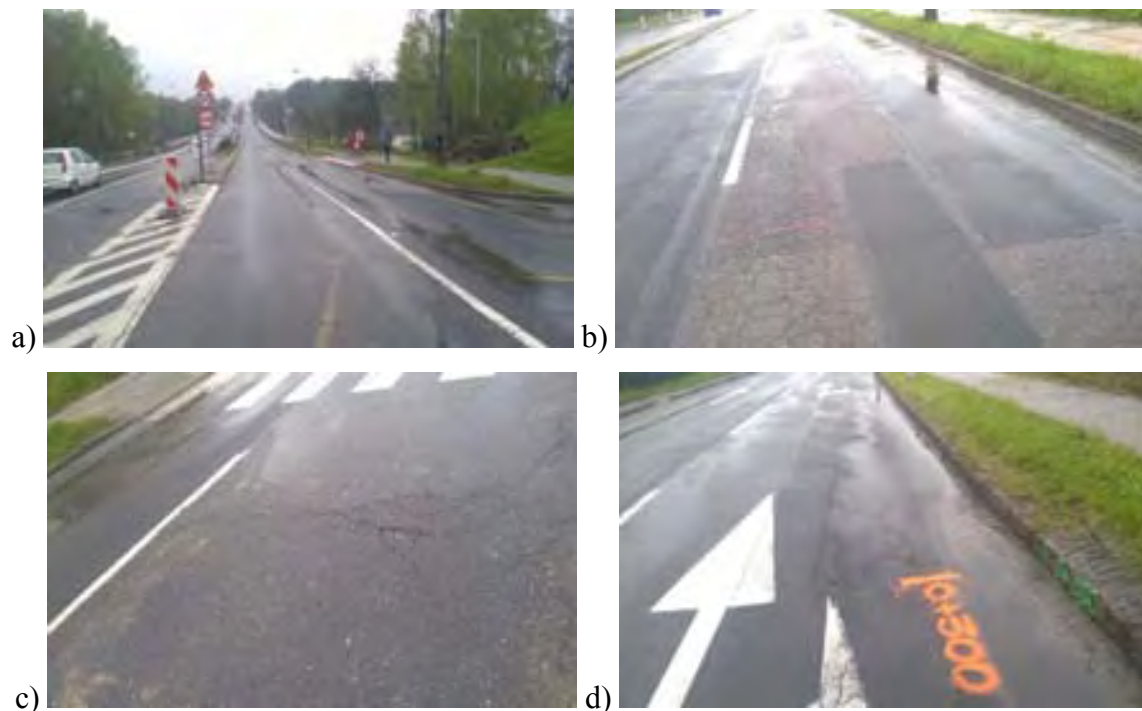
Figure 2. Fragment of Matuszczyka Street in Wodzisław Śląski a) general view, b) mesh patches and cracks in the pavement, c) transverse crack, d) longitudinal crack (own elaboration).
