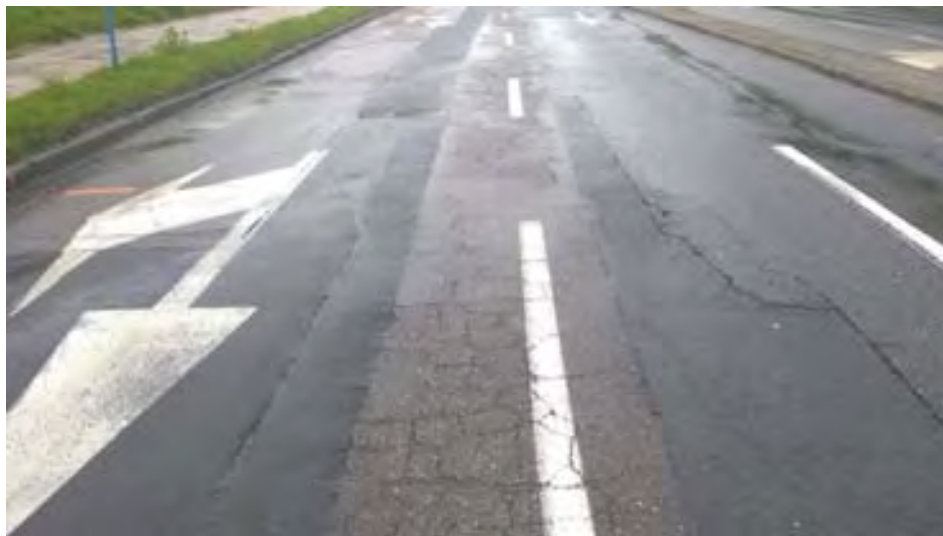
Figure 3. Patches and cracks on the section (0 + 300 - 0 + 400) of the tested road (own elaboration).
