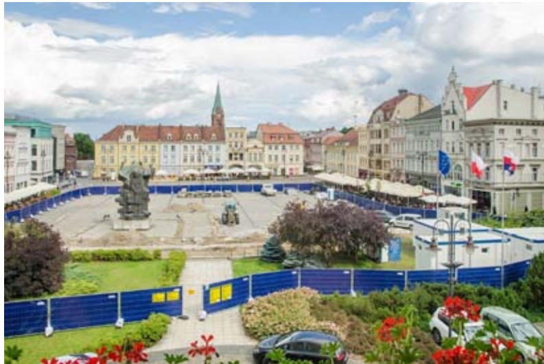
Figure 1. Revitalization works on the Old Market Square in Bydgoszcz. Source: Bydgoszcz w Budowie [Bydgoszcz under construction – Old Market Square] website, Beginning of revitalization, 22.10.2021.
