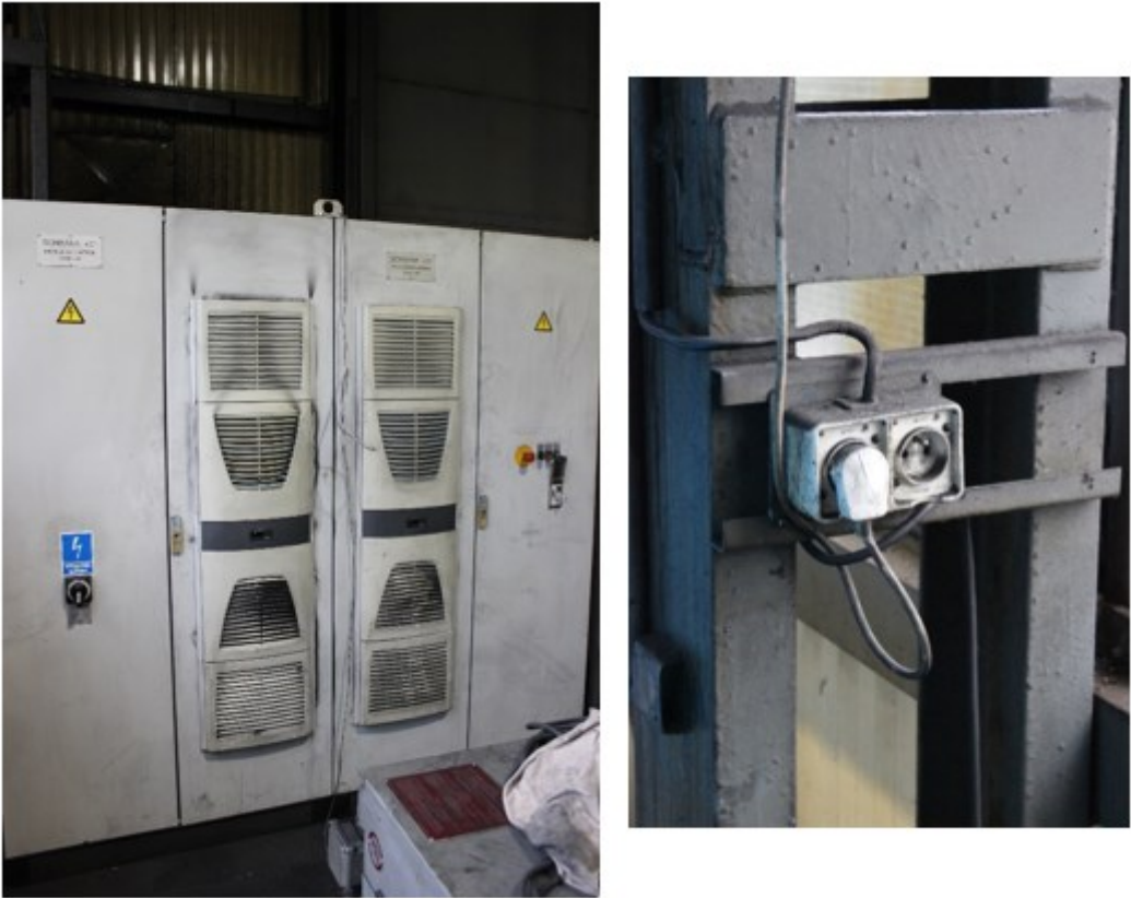
Figure 2. Dirt on the cabinet, electric cable filters and 220V sockets.
